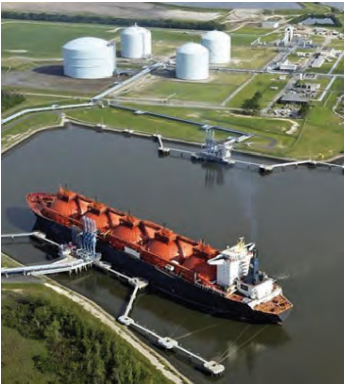
Insulated Low Pressure Storage Tanks for LNG
